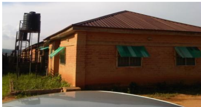
Figure 3. Sample Unit of Nigerian Army Retired Officer's Quarters showing material of wall construction
